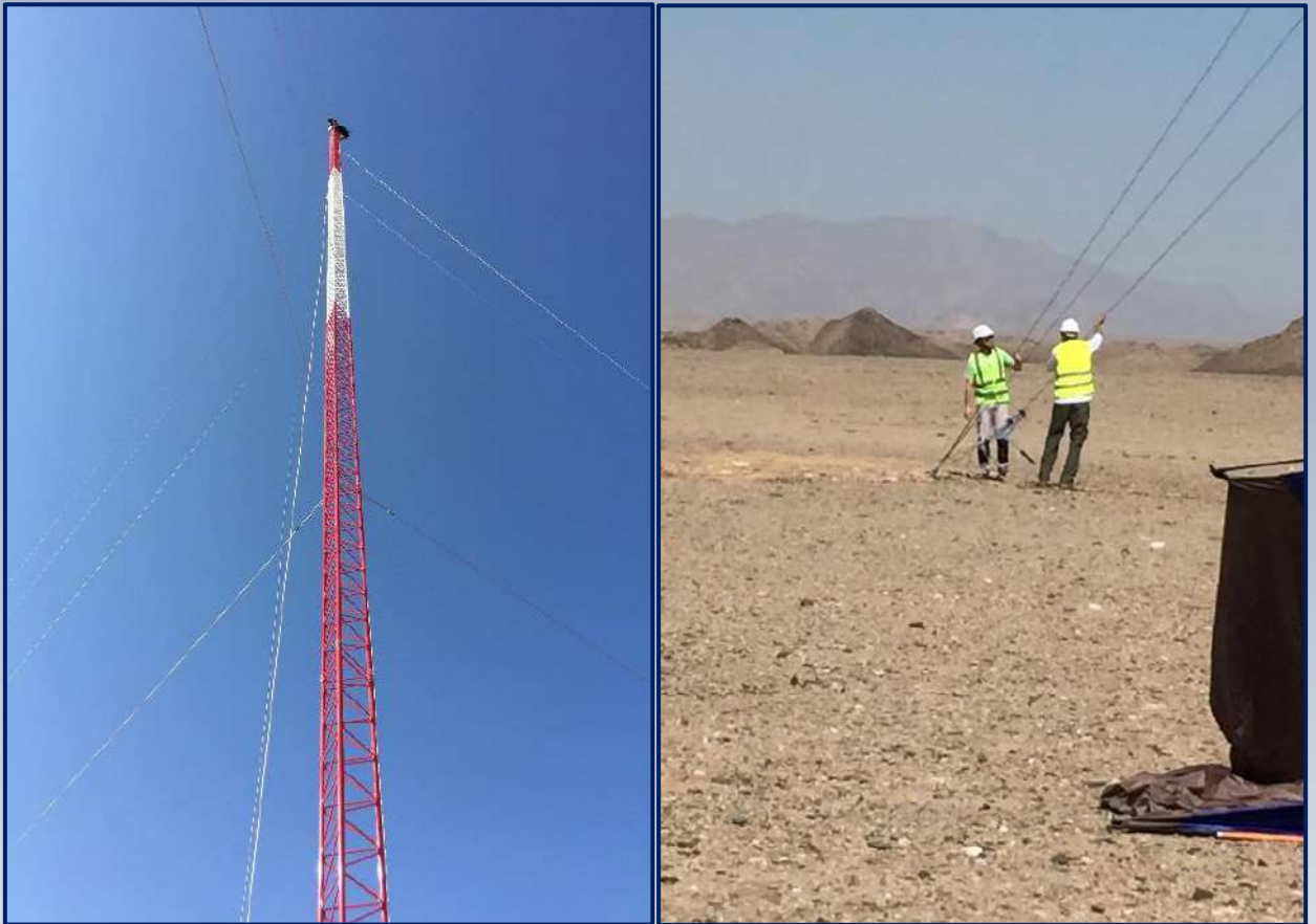
Figure 3: Installation of Anchors
