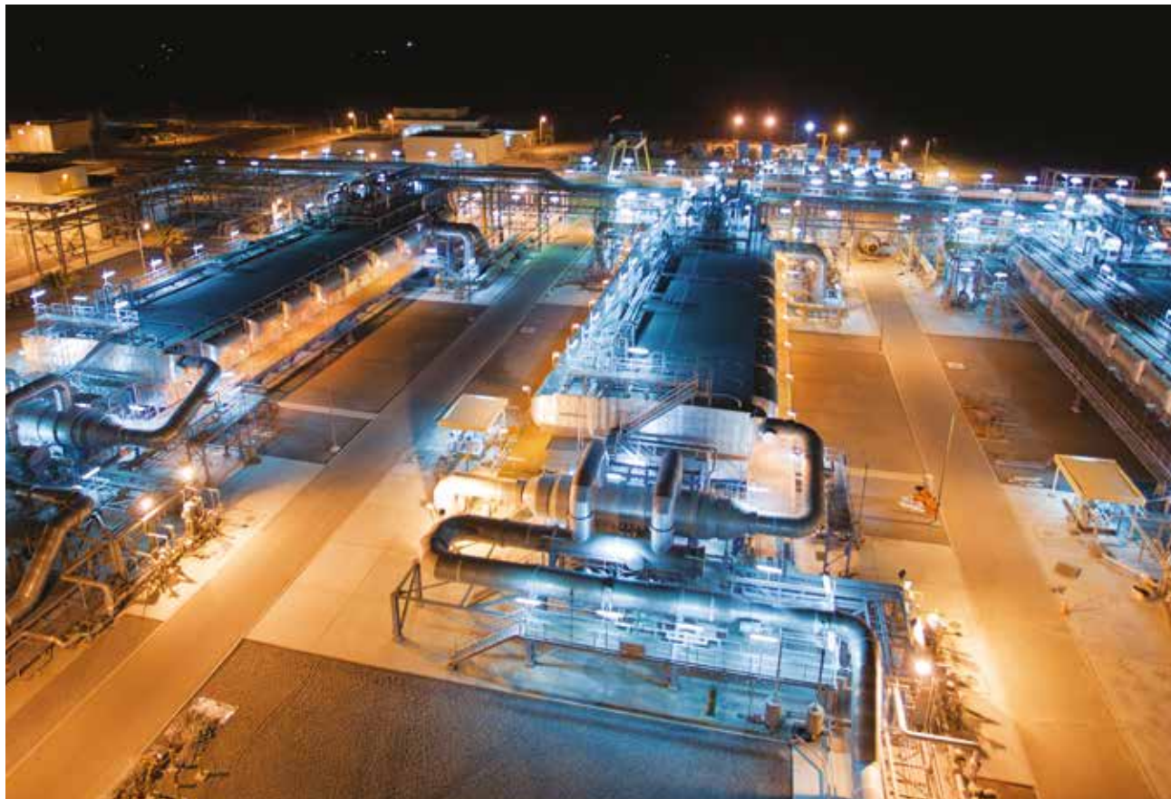
— Barka I Power and Water Desalination Plant
