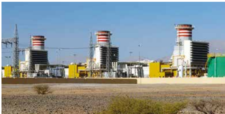
— Al Kamil Power Plant
