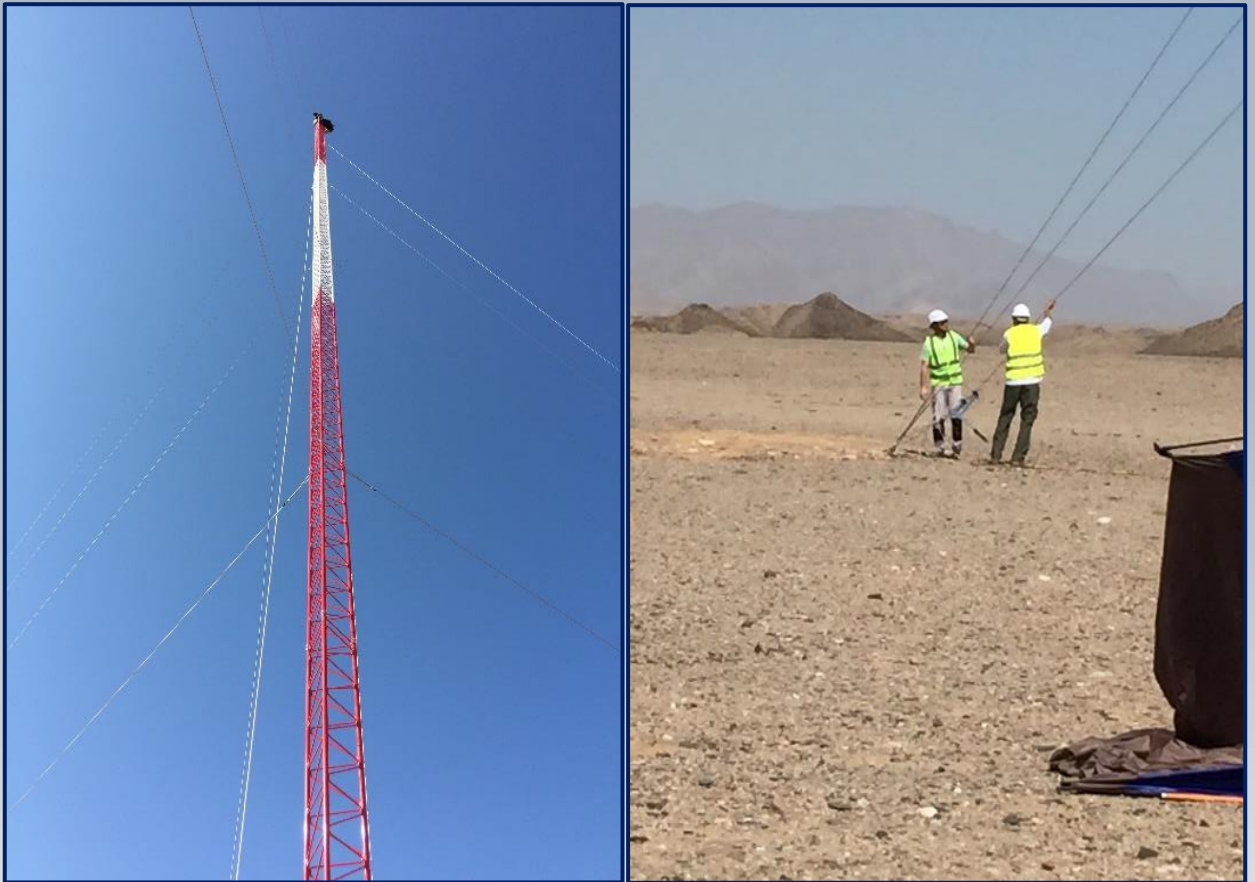
Figure 3: Installation of Anchors
